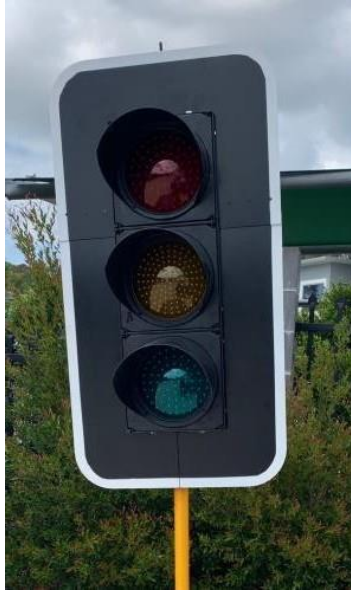
FIGURE 18 – Target board installed
